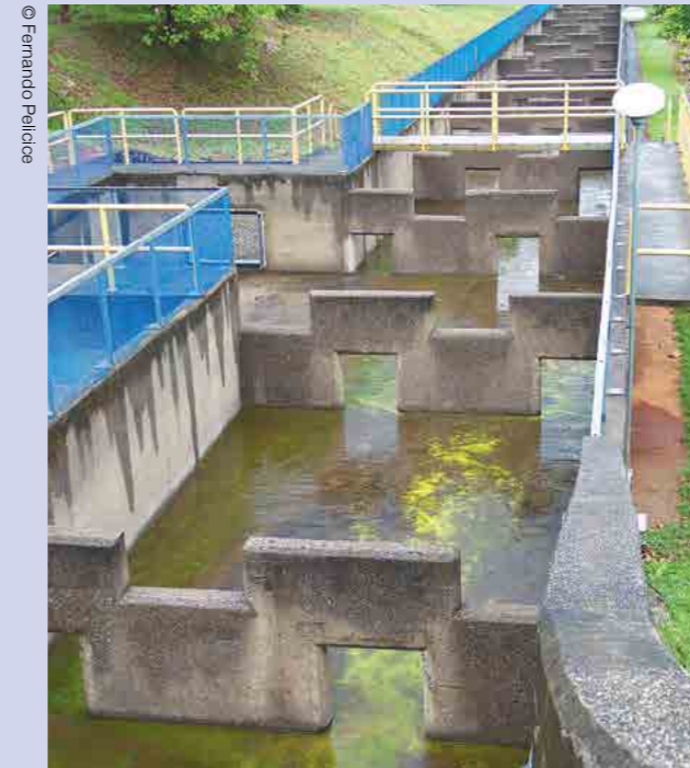
Fish ladder at the Lajeado dam was closed. Studies have proven that such mitigation actions have failed to preserve fish migration.
