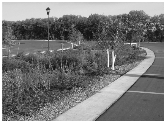
FIGURE 13. A bioretention cell, such as the one pictured here, contains a specially designed substrate and vegetation, typically native plantings, that can absorb and filter runoff from adjacent impervious surfaces. (Photo courtesy of the USDA Natural Resource Conservation Service.)
